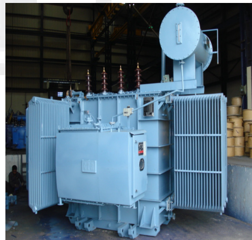
6.25 MVA Power Transformer for Jyoti Sugar Ltd.
