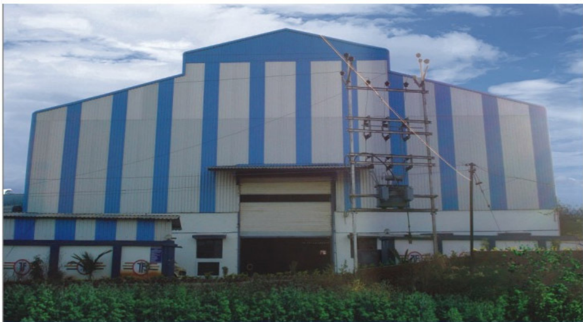
Front View of Factory
