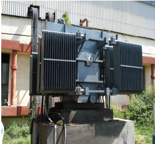
4 MVA Transformer Manufactured and Installed at Vaidhynath Sahakari Sakhar Karkhana
